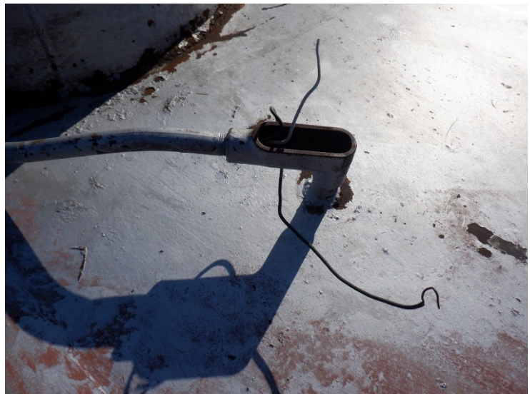
47) There is exposed wiring at a damaged junction box on the roof.
