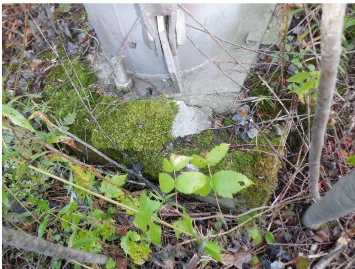
12) There is missing grout between the steel leg baseplates and concrete foundations.
