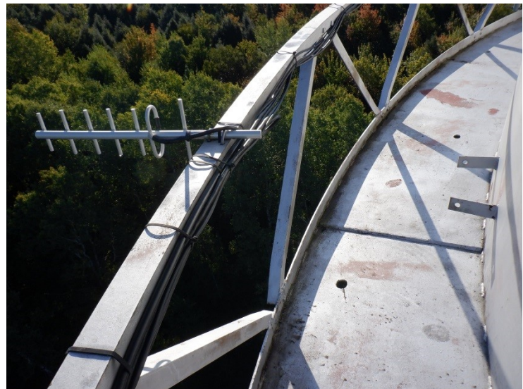
35) There are numerous coating failures on the balcony.
