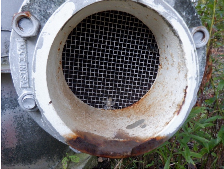
25) The screen at the overflow pipe discharge is intact but oversized.
