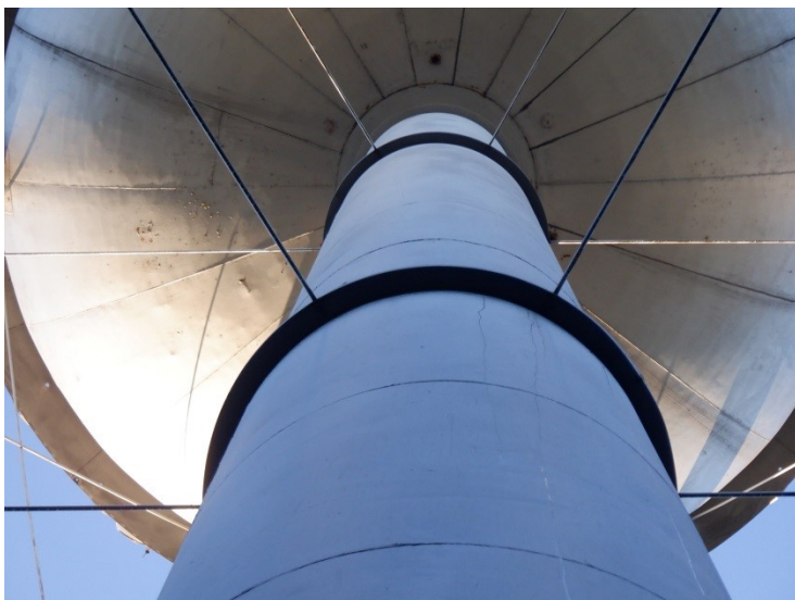
9) The riser tie rods are in good condition.
