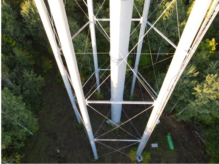
22) The sway rods are in good condition.
