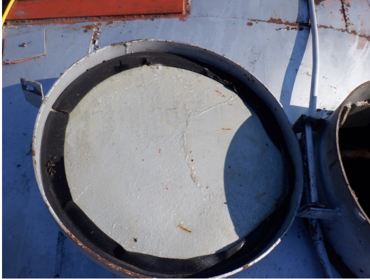
46) There is a gasket on the wet interior roof hatch.
