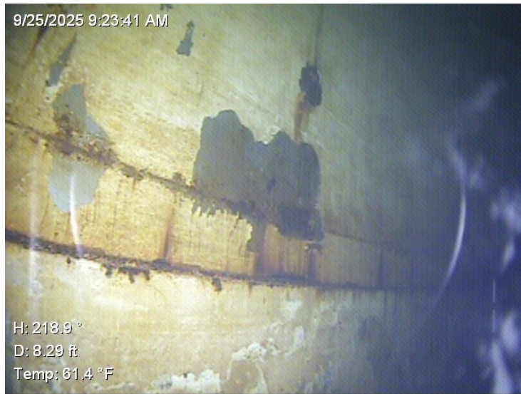
67) The wet interior sidewall coating is in poor condition with extensive failures.
