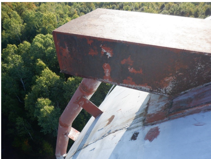
48) The roof coating is in poor condition with numerous failures.
