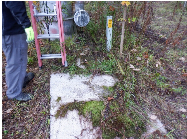
23) The overflow pipe discharges to a concrete splash pad.
