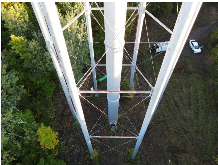
21) There are coating failures on the struts.
