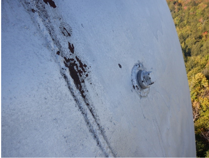
55) The roof rigging couplings are properly capped.
