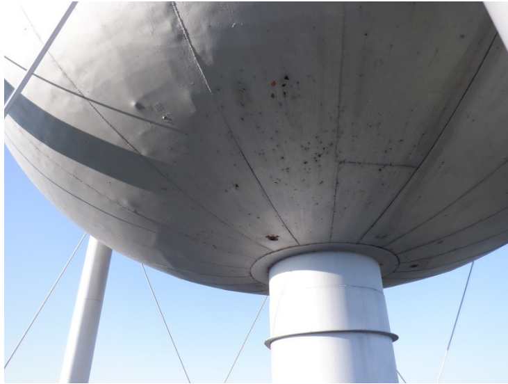
28) The bowl coating is in fair condition with a few failures.
