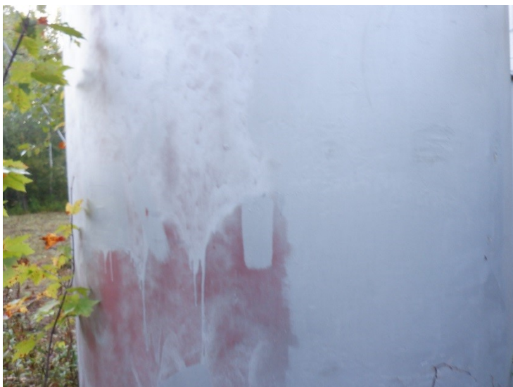
6) There are a few coating failures on the riser.
