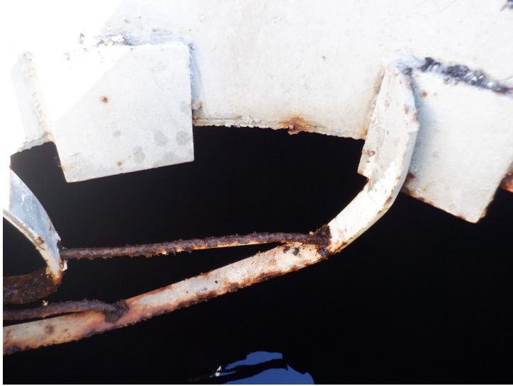
61) There are remnants of an old damaged wet interior ladder.
