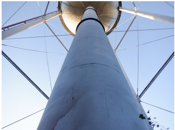
8) The riser coating is in fair condition overall.
