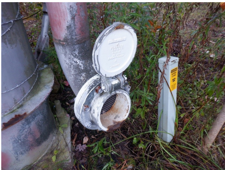
24) The solid flap gate at the overflow pipe discharge operated properly.
