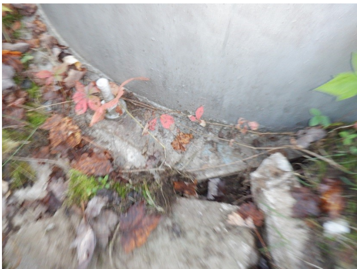
3) The concrete riser foundation is in good condition with no significant deterioration.
