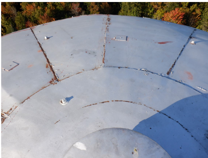
54) The cathodic lift holes on the roof were found to be properly aligned.
