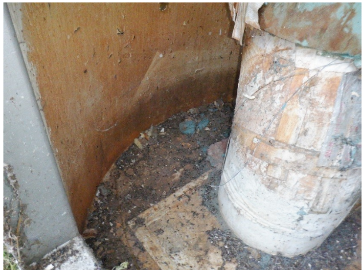
59) The expansion joint on the bottom of the fill/draw pipe in the riser is covered with insulation and not accessible for inspection.
