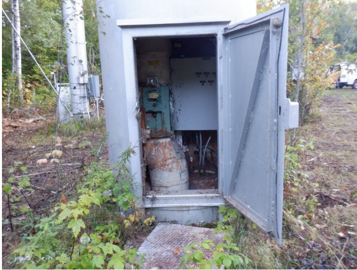
58) The service door in the riser operated properly. There is no ladder in the dry interior riser.
