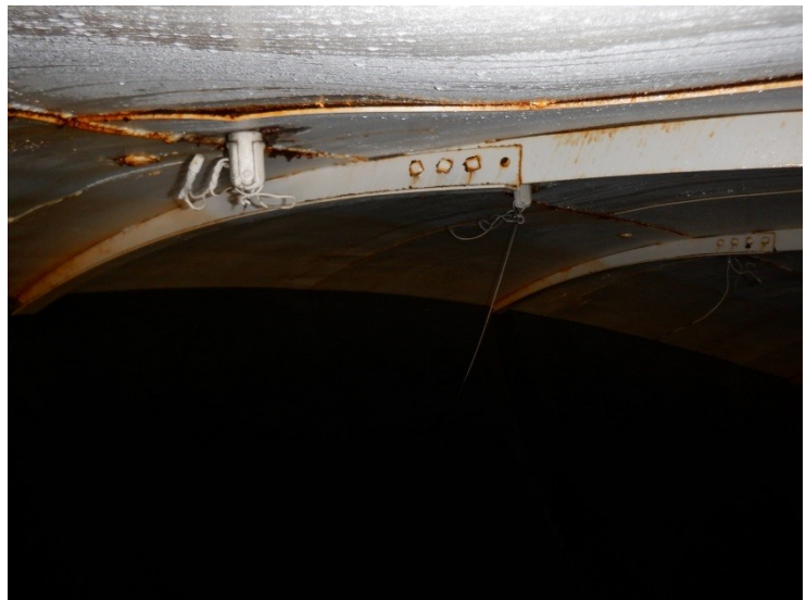
62) The wet interior roof coating is in poor condition with numerous failures.
