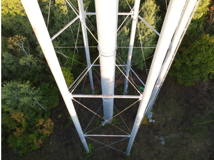
19) The leg coating is in fair condition overall.
