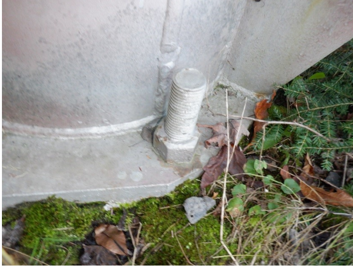
13) The leg anchor bolts are in good condition.
