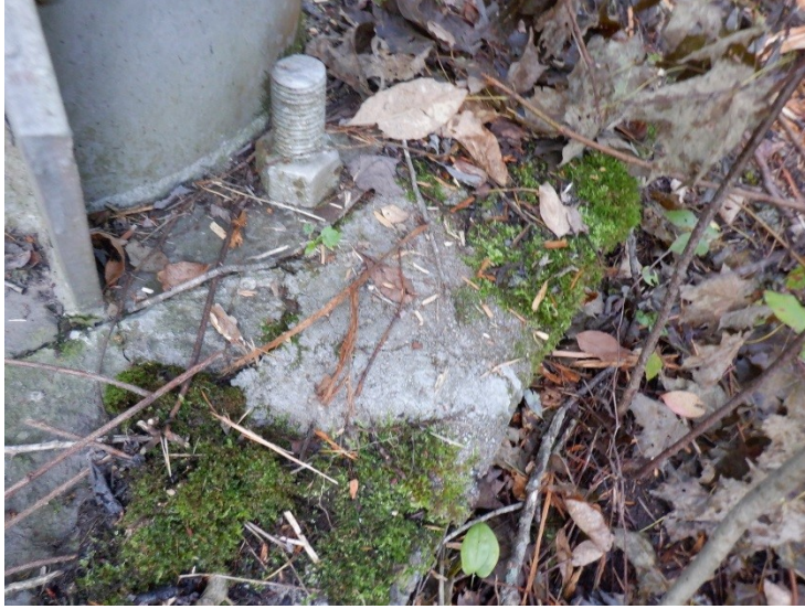
10) The concrete leg foundations are in fair to poor condition with moderate deterioration.
