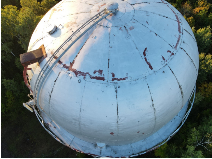
43) The sidewall/roof ladder is in good condition.
