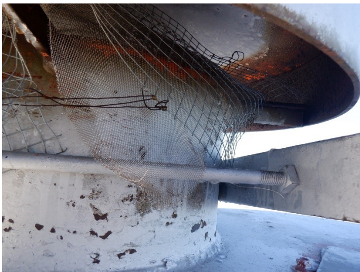
57) The roof vent screen is damaged.
