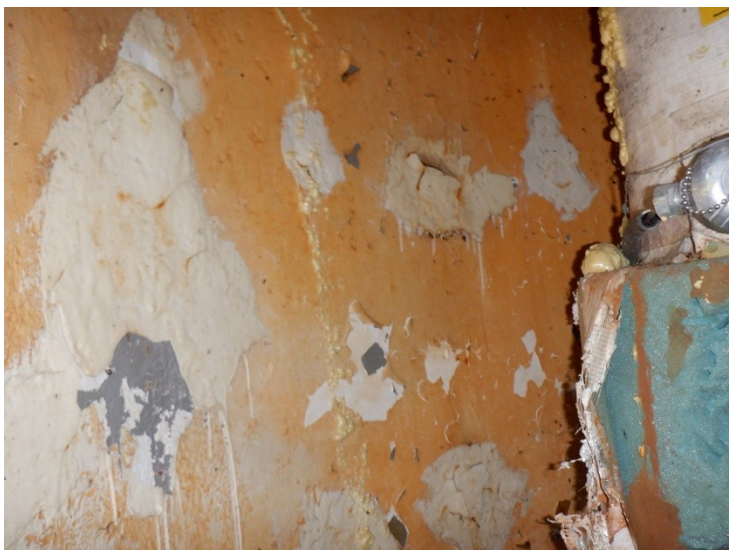
60) The dry riser coating is in poor condition with numerous failures.
