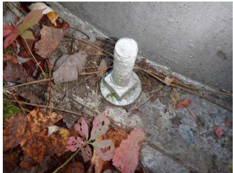
5) The riser anchor bolts are in good condition.
