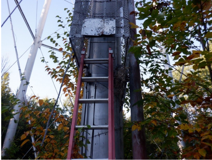
1) Tree branches and vegetation are rubbing and encroaching on the tank.
