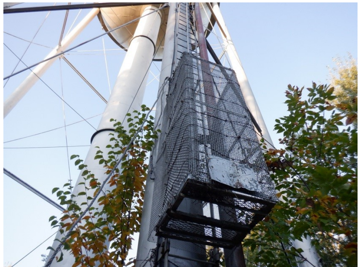
26) The vandal guard on the leg ladder is in good condition.
