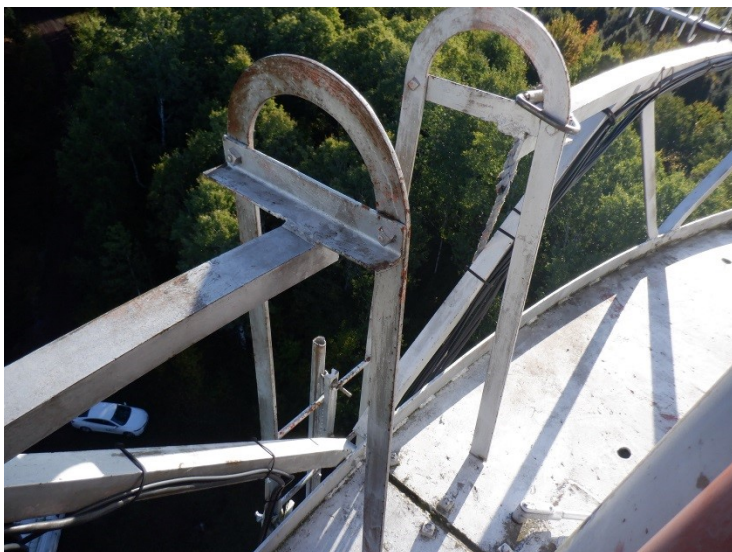
33) There is not a swing gate across the leg ladder opening in the balcony railing.
