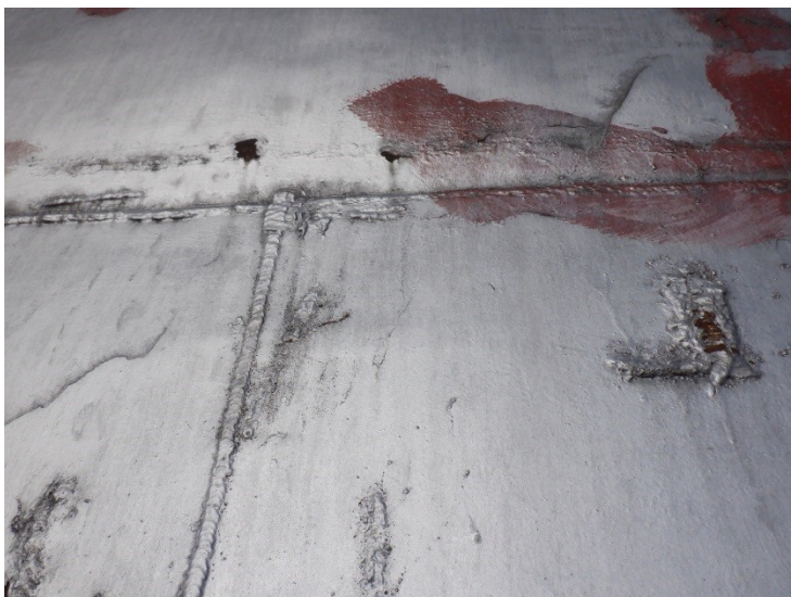
36) The sidewall coating is in poor condition with numerous failures.
